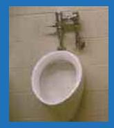
University of Washington: Non-Zurn 0.5 GPF urinal system. Notice the alterations made in the piping in order to fit the footprint.
