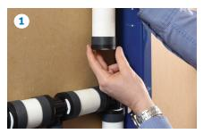
Fully insert piping into QickCap Copper Crimp Ring.
