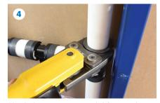
Crimp the ring to create a permanent, leak-free connection.
