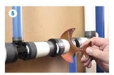
Use gauge (large diameter Go-Go Gauge, QGA678CR shown) to verify that a secure crimp has been made.
