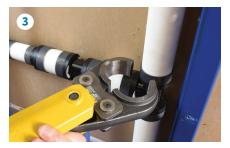
Open jaws of crimp tool (QCRBTKIT56-14V power tool shown), and place over properly aligned QickCap crimp ring.
