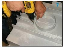
7. Once outlet is placed, attach outlet with supplied screws.
