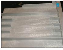
5. Rough fit out onto basin, ensuring there are no obstructions and outlet seats flush.
