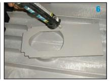
6. Apply construction adhesive to outlet and place in required position.
