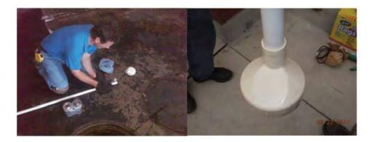
Cut  $\frac{3}{4}$ " PVC pipe to length (A +  $\frac{1}{2}$  B) so probe end is positioned in the middle of the interceptor liquid level. Run the black wire from the probe through the PVC pipe. Secure probe to the PVC pipe with PVC cement to create a waterproof seal.
