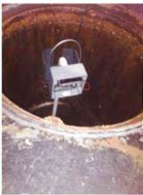
Remove cover from back of control box with 4 screws. Place probe through U-bracket and into interceptor until control box elbow rests on bracket (this is actually inserting the probe backwards at this point).
