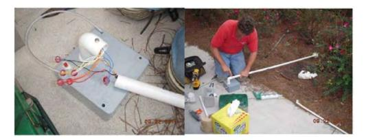
Remove the set screw from the control box elbow and push the connectors down into the ¾" pipe and up into the ¾" elbow. Put a bead of **100% silicone rubber** on the outside end of ¾" pipe and push pipe into the elbow until seated. Rotate the probe end so that when the control box is inserted into the bracket and the probe end is in the tank, the probe end is not facing a wall, pipe or any other obstruction and then install the set screw into the ¾" elbow.
