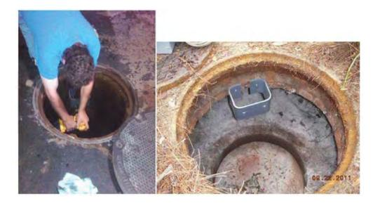
Install U-bracket level in manway riser with 2 mounting bolts provided. Bolt holes should be drilled into the riser approximately 15" from grade in a position where underwater probe does not have obstructions and the manway cover will not interfere or damage the control box.
