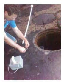
At top end of PVC pipe, cut black wire approximately 6" longer than PVC pipe. Strip black wire shielding to expose wires but do not strip individual wire jacketing.
