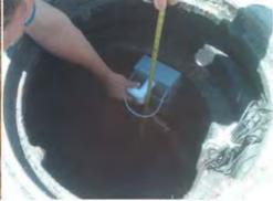
Insert control box into the U-bracket as shown. Measure the distance from the ¾" PVC elbow (with 6 wires) to the top of the grease layer/liquid level (Dimension A). Then measure the liquid level to the bottom of the tank (Dimension B) [See Figure 1]. Tank bottom must have no sediment build-up to insure accurate measurement.
