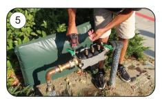
Remove Flush Fitting Tool and reinstall EZSwap™ Pressure Vessel.
