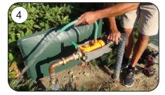
Turn on inlet ball valve, direct water to landscaping or safe drain, and flush until clear
