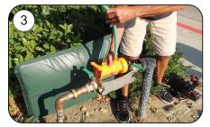
Drop in and install Flush Fitting Tool. Attach hose.
