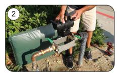
Un-bolt and remove EZSwap™ Pressure Vessel.
