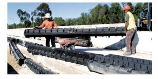
Z888-12/18 Hi-Cap® Drain System With Transition Piece
