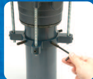
Tighten to pipe with allen wrench.
