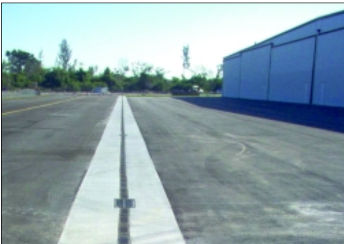
Airport Trench Drain
