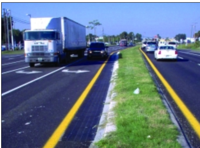
Median Trench Drain
