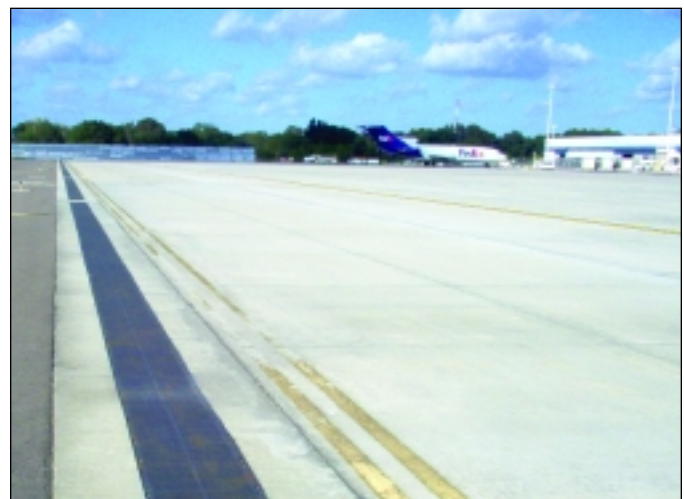
Airport Trench Drain
